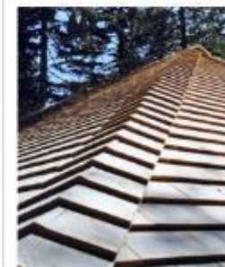
Roof Shingles & Shakes
